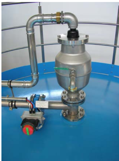
Sample installation on oxidizer tank
